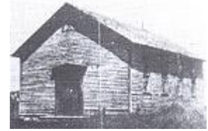
Church of St. John the Baptist also known as the French Catholic Church built in 1868 on Adolph Crevier's property.
